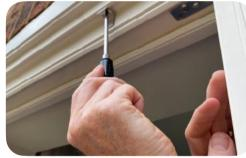
2-5m. The clips can be fixed vertically or horizontally. Screw the 2 mounting clips about 25-45cm apart (depending on which length light) to the wall (or overhang) with the supplied screws.
