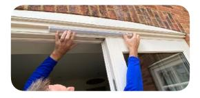
The distance between the clips isn't critical as they can fit on anywhere along the length of the aluminium part of the light. To mount the light simply fit one edge into the top or bottom of the clips then twist it round until it clicks into place. The cable should be routed indoors or connections made in a weather-proof junction box. Recommended maximum cable run between the power supply and the light is 50m when using 0.5mm cable.
